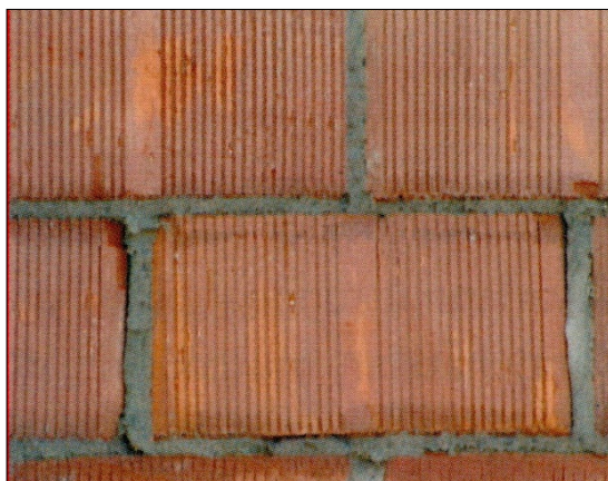
Figure 101 Proper Application of Plaster in Both Directions
