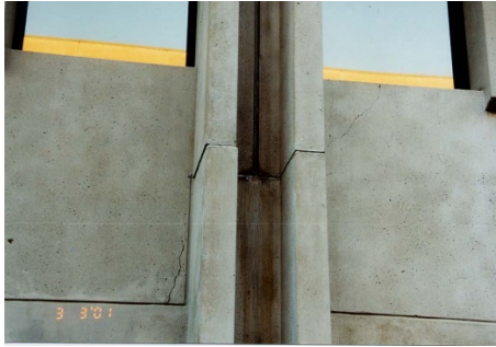
Figure 113 Crack Near a Window
