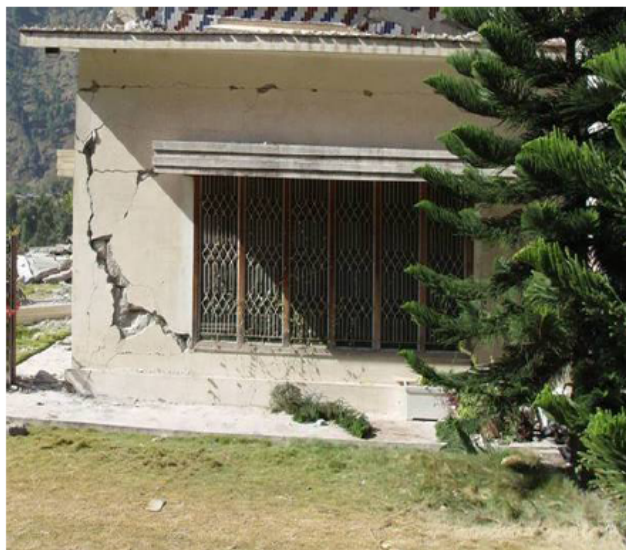
Figure 120 Damage Grade-3 (Masonry Building)
