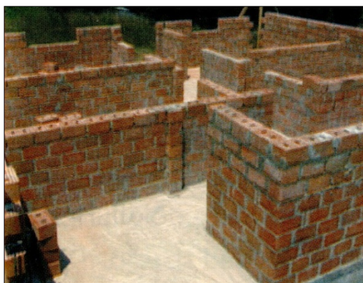
Figure 103 Proper Construction of Load Bearing Walls
