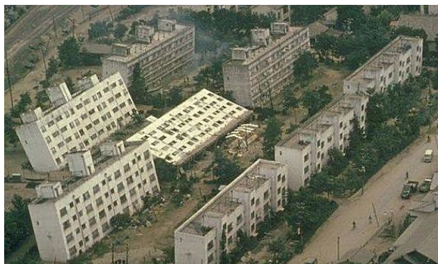
Figure 46 Permanent Displacement Caused by Liquefaction Following the Earthquake in 1964, Niigata, Japan
