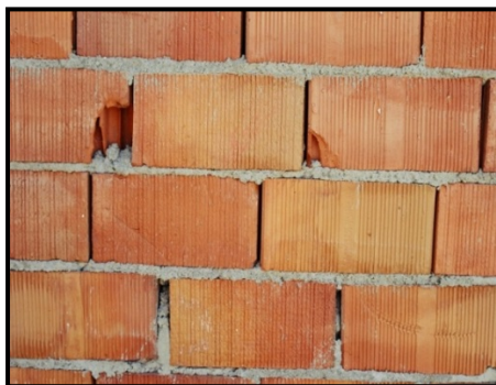
Figure 102 Improper Application of Plaster and Low Quality Brick
