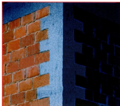
Figure 87 Connection of Two Load Bearing Walls at the Corner
