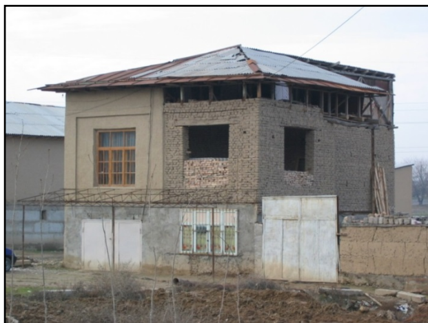
Figure 96 Openings of Load Bearing Walls Which Exceeds Limit
