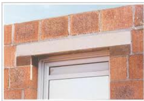
Figure 79 Horizontal Lintels over a Window
