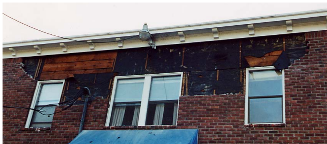
Figure 114 Damage in Roof Zone
