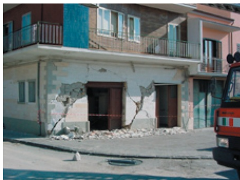
Figure 112 Shear Failure - “X” Shape Cracks
