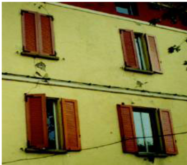
Figure 118 Damage Grade-1 (Masonry Building)
