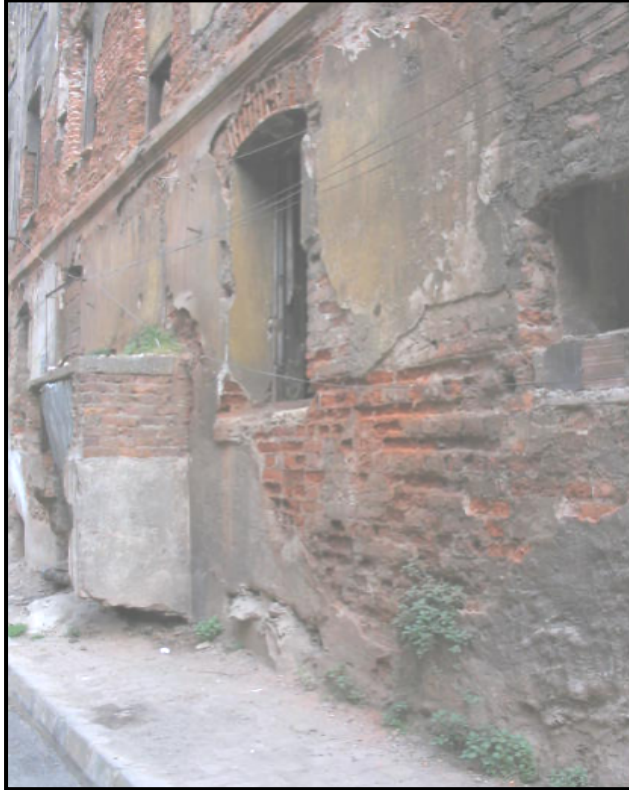
Figure 105 Deterioration of Load Bearing Walls due to Water
