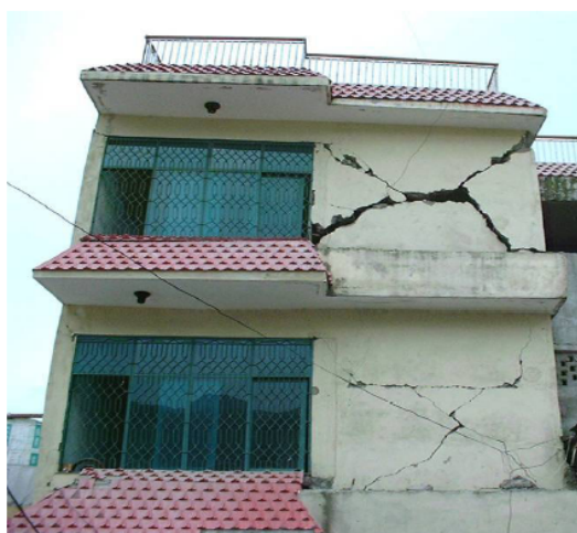
Figure 121 Damage Grade-4 (Masonry Building)
