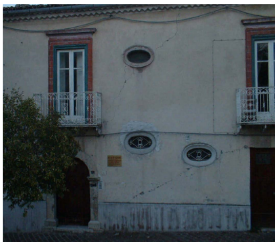
Figure 119 Damage Grade-2 (Masonry Building)
