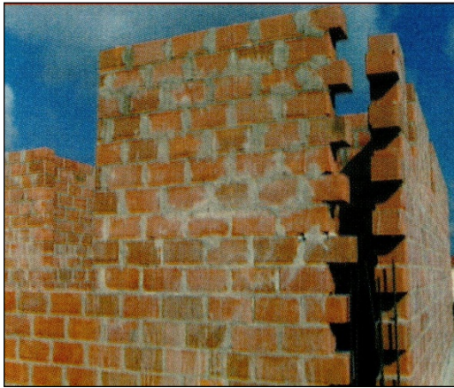
Figure 91 Vertical Lintel Application
