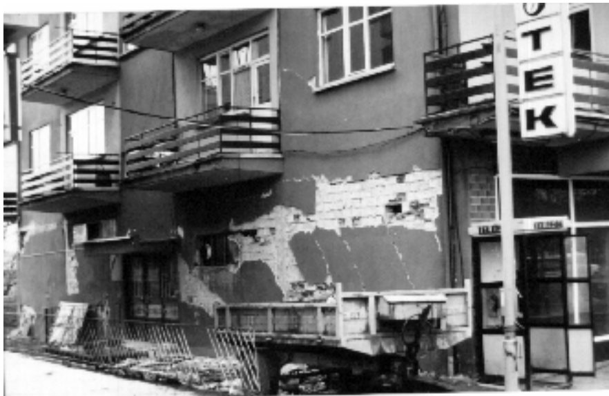
Figure 6. Failure of the infill in a building (Erzincan Earthquake).
