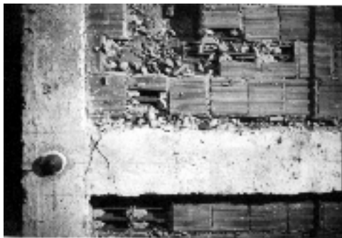
(a) Nonplastered Infilled Frame
